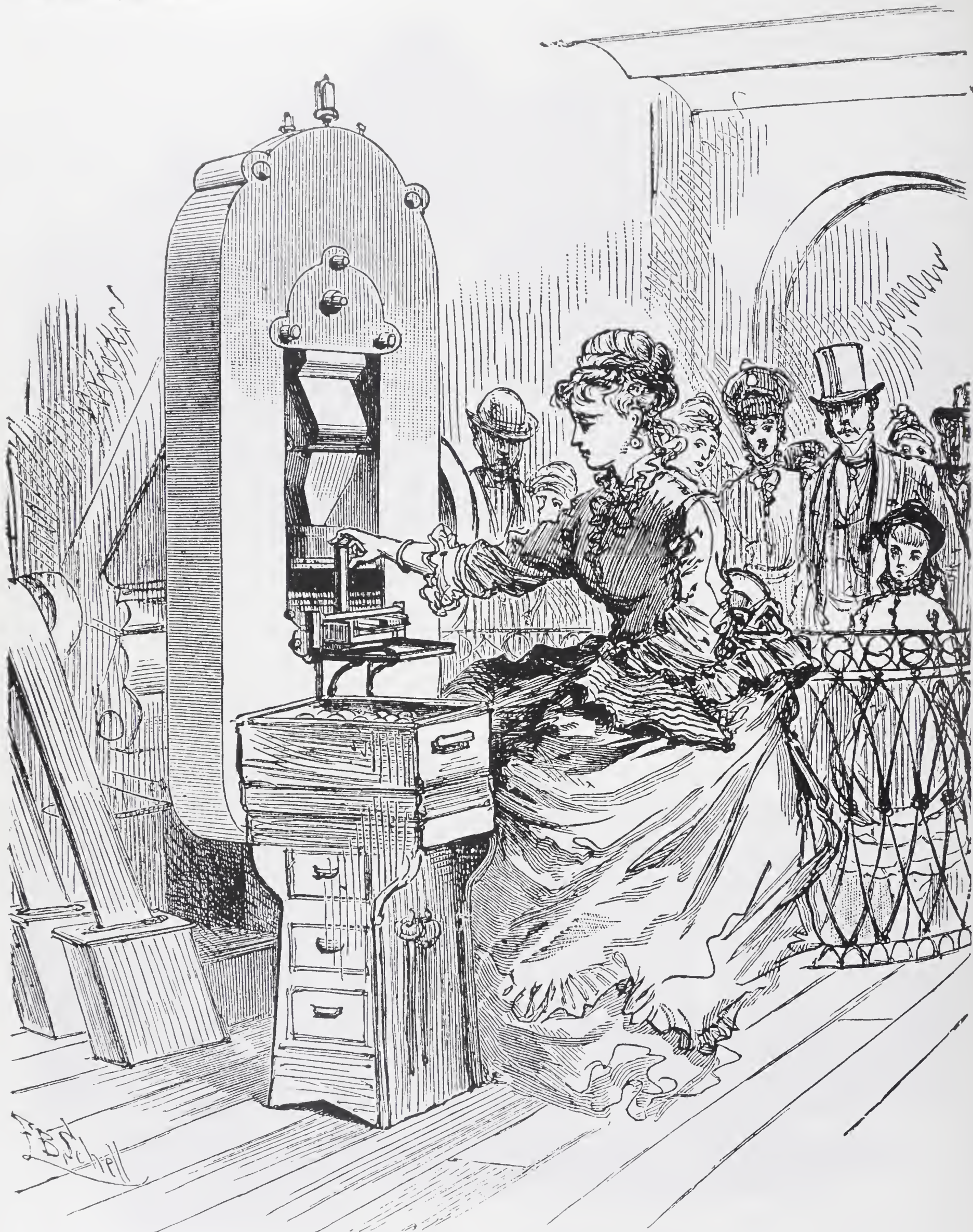
Operating a steam-powered coining press at the Philadelphia Mint, circa 1853.
